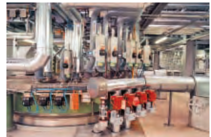
At the Deutsche Shell AG in the plant Grasbrook over 2,000 valve actuators are networked via the AS-i interface.
