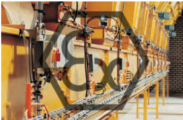
ClassicLine modules for field applications in hazardous areas.
